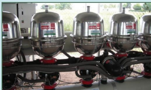
In technology from Israel, a series of sand filters cleans water for use in drip irrigation.
