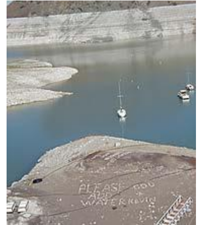
Low Water Levels at Elephant Butte, Courtesy of Bureau of Reclamation 135
